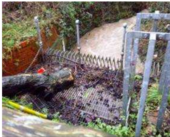
Figure 3.8: Black Ditch Culvert – Feb 2014
